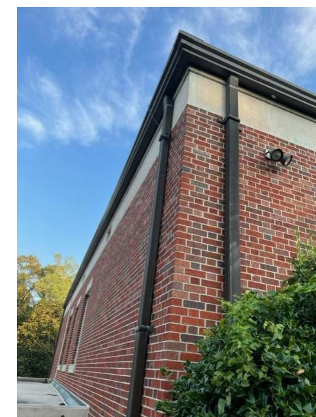
(H) REMOVE AND TURN OVER TO THE OWNER EXISTING COPPER GUTTER AND DOWNSPOUT SYSTEM.
